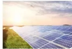
Energy Storage System
