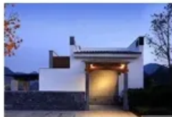
Household Energy Storage
