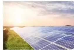
Energy Storage System
